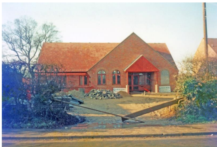
February 1989 "The Daisy" Under Construction
